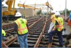
Rail system rehab
